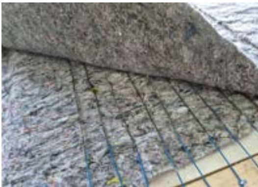
Fig. 28 Self Regulating Heating Cable
