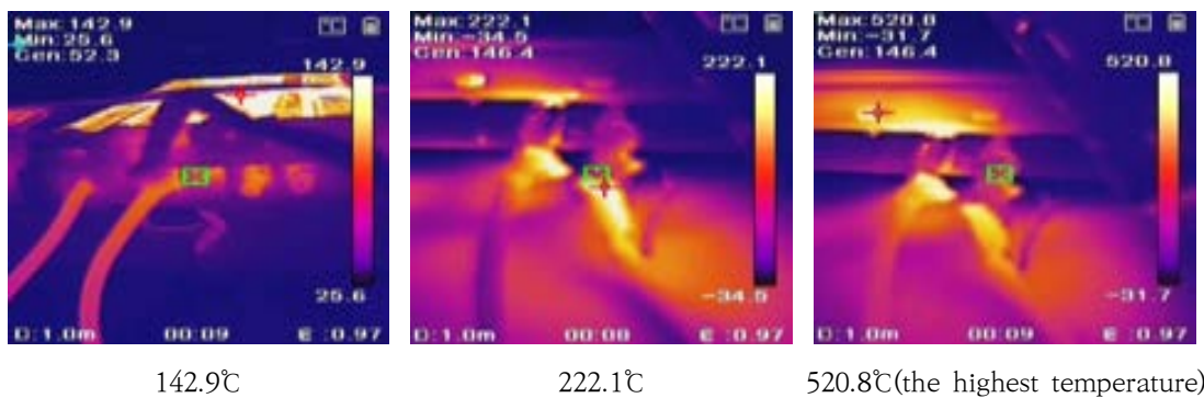
Fig. 12 Measurement of temperature change at ptc connector connection terminal
