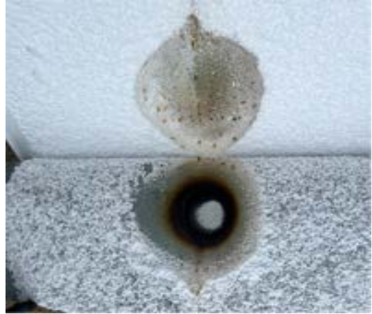
Fig. 10 Inside the sandwich panel.
