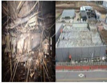
Fig. 6 Roof and a second floor.
