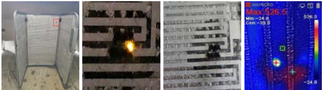
Fig. 28 Silver Busbar Damage (B사)
